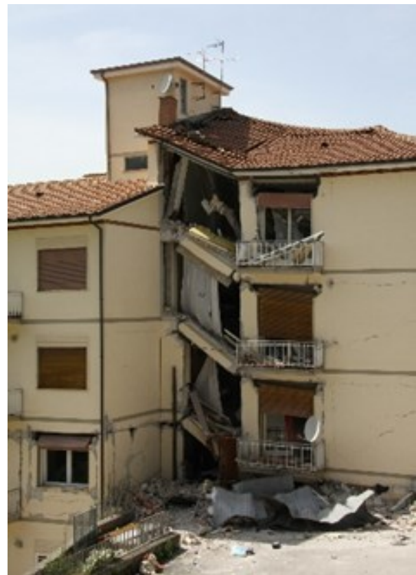
Partial collapse of a residential building after the 2009 L'Aquila earthquake
